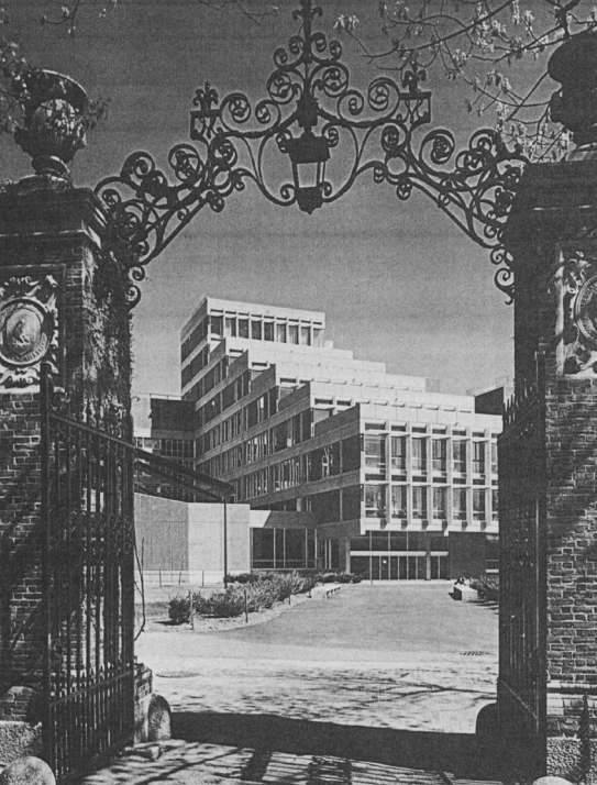
Newly constructed Science Center.
